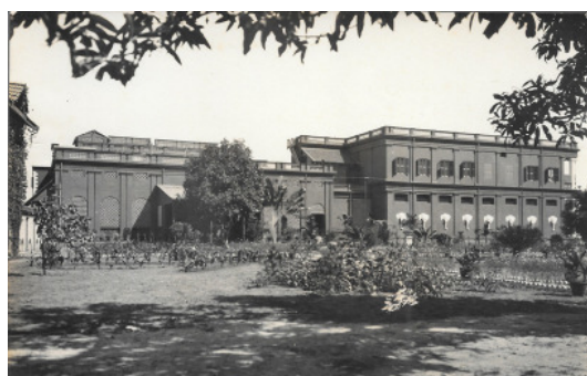
The Headquarters building after the installation of the eight bas-relief elephant heads
