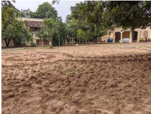
Removal of the existing top soil on the lawn
