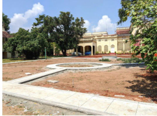
Laying of the granite pathway
