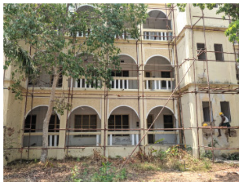
Leadbeater Chambers under renovation
