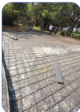
The new concrete road being laid (2026)
