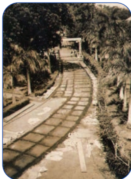
The old concrete road being laid (1937)
